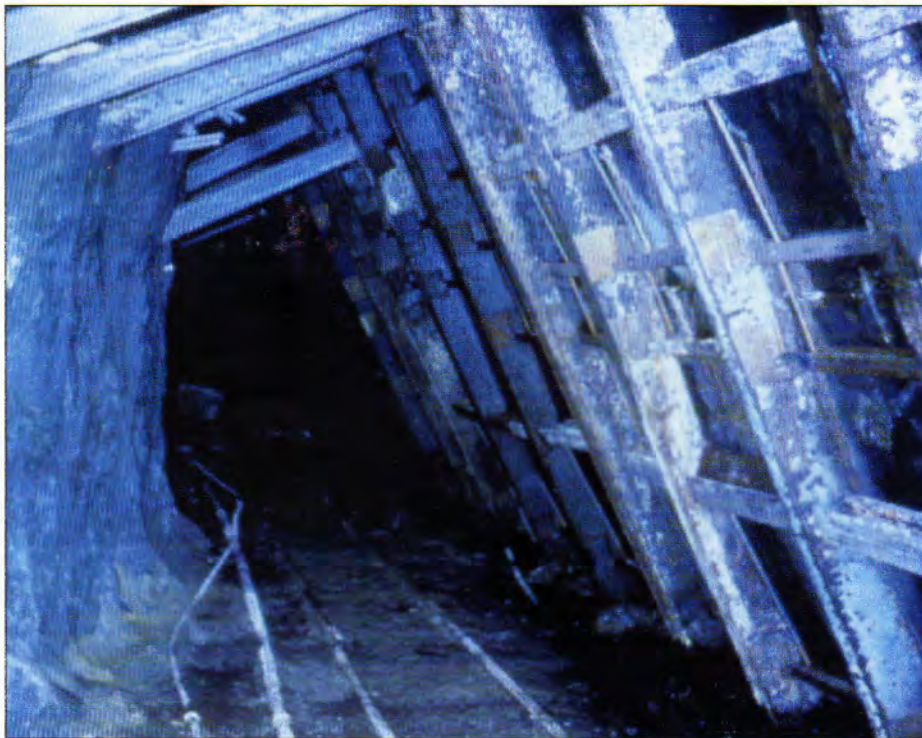
Old steel sets in a mined out and abandoned part of the Sterling Hill mine, circa 1976. F. Bernard Kozykowski archives photo.
