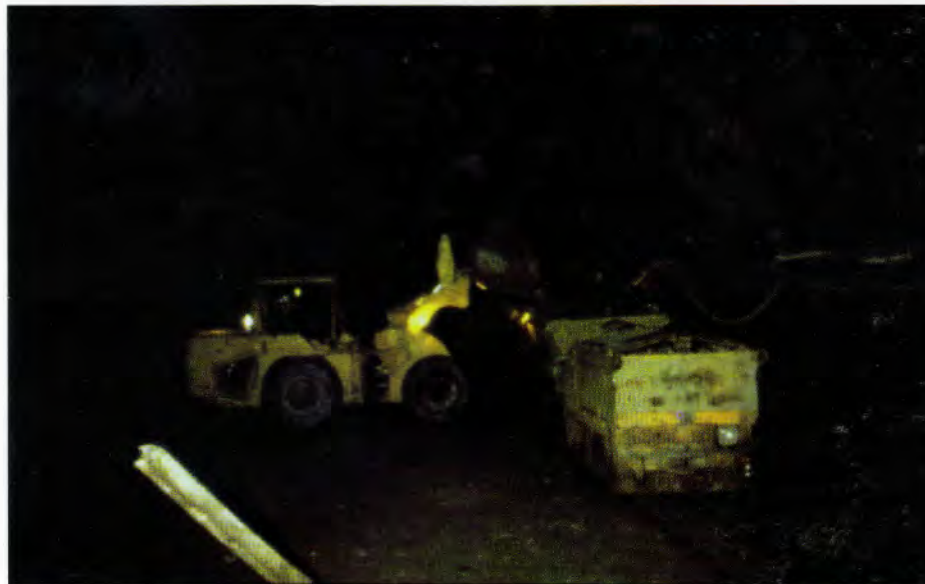
Eimco LHD loading an ore car. Sterling Hill, circa 1976. F. Bernard Kozykowski archives photo.
