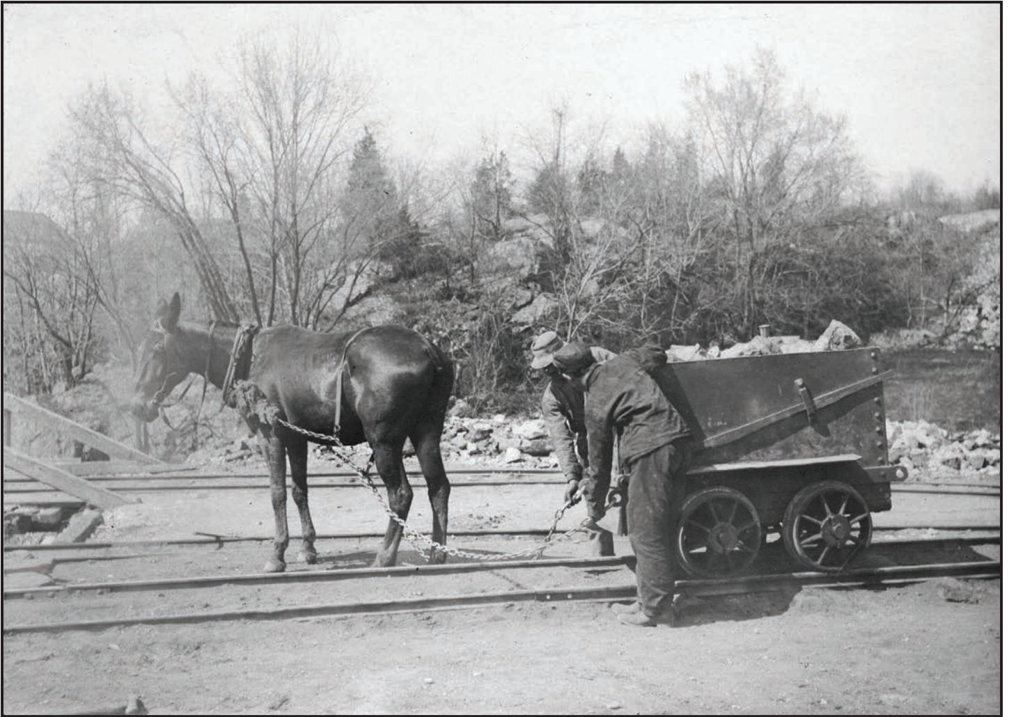
Tramming waste rock via horse-drawn car on the Buckwheat Dump during the period of the operation of the Taylor Mine, circa 1890s. View is looking toward the west. This photo is from an album in the archives of the Franklin Mineral Museum.
