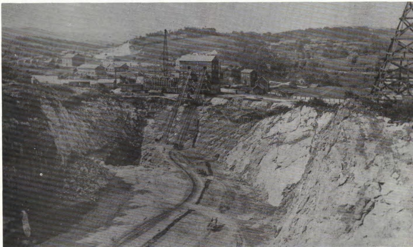
*Figure 6.* The Buckwheat Open Cut showing mule wagons, inclined rail tram, aerial tram, and mill, 1906.
