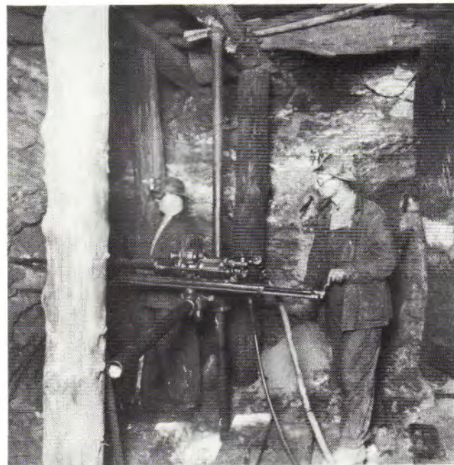
Figure 2. Drilling a round in the Franklin Mine, Franklin, New Jersey, circa 1930-40. Photograph courtesy of Bob Svecz and the Franklin Mineral Museum archives.
