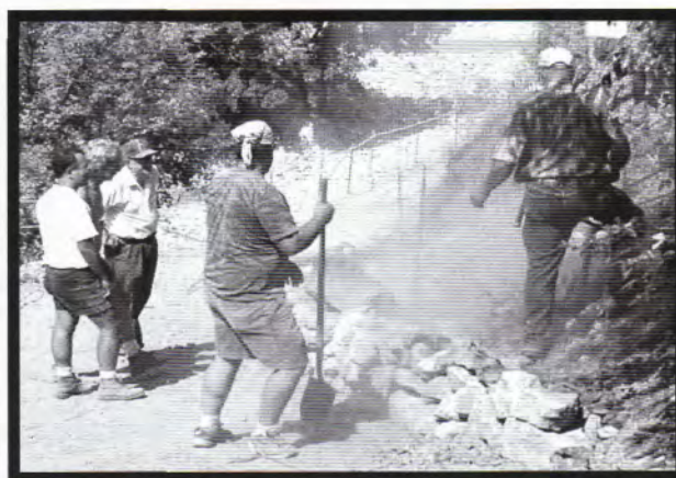
FOMS volunteers building a retaining wall on the new "Buckwheat Trail"
