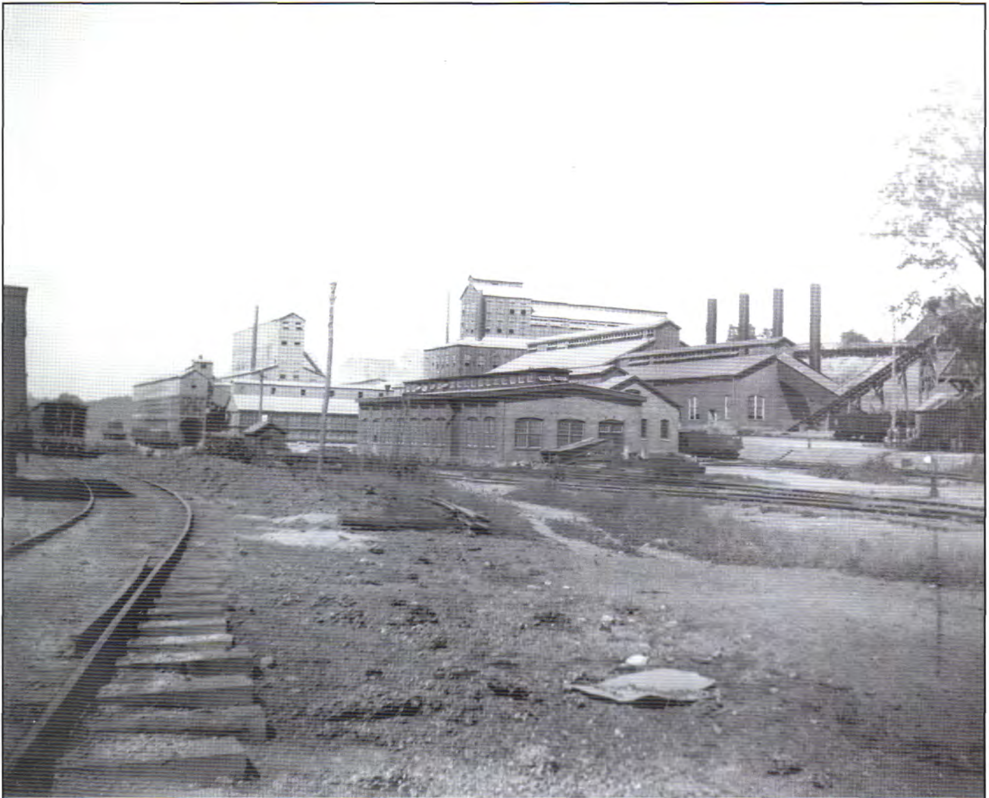
Franklin Mill No. 2, which went into service in 1900 to treat the ores coming out of the Parker and Trotter shafts. This scene was photographed on July 11, 1908. Notably absent in this early view of the mill is the Palmer Shaft hoist and ore conveyor, which would distinctively mark the Franklin skyline within two years. In the foreground is the machine shop; to the right was the shed where the plant's lubricating oil and grease were stored. The building next to the four smokestacks is the boilerhouse for the power plant that provided electricity to the consolidated Franklin mining operations. When the Palmer Shaft began production, this mill complex was substantially expanded and became known as the Palmer Mill.
