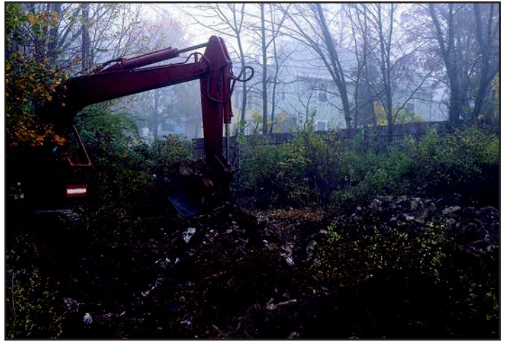
Figure 4. Excavation begins - October 1984.
