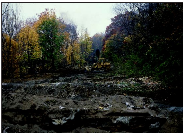
Figure 6. Stripping away the overburden from the trestle.
