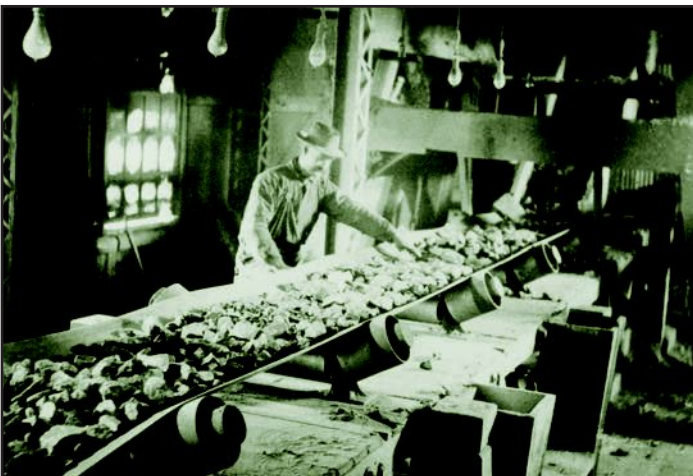
Figure 1. Conveyor at the headworks of the Parker Shaft. Photo from Franklin Mineral Museum archives.
