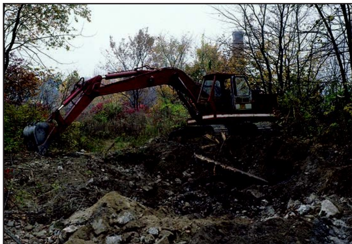
Figure 5. The first trestle timber is encountered - note the bracket arms.
