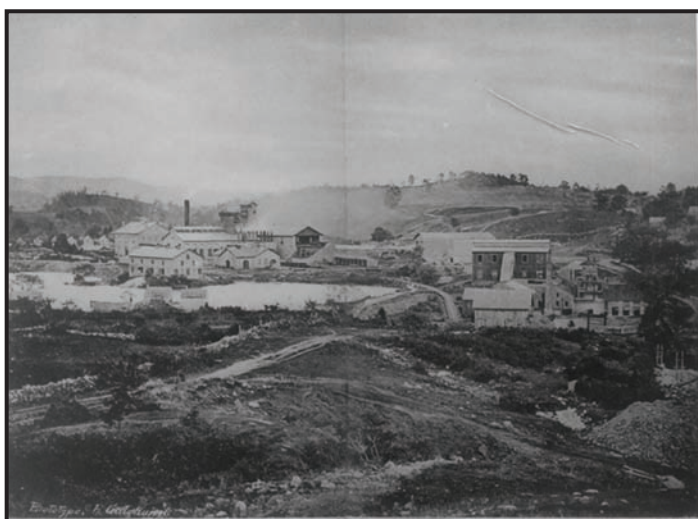
Figure 4. Late 1800s blast furnace in Franklin.
